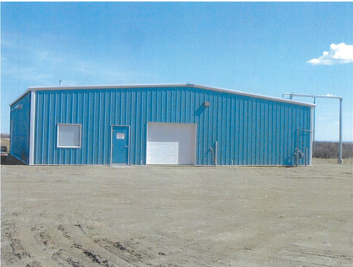
The Melita Water Treatment Plant
